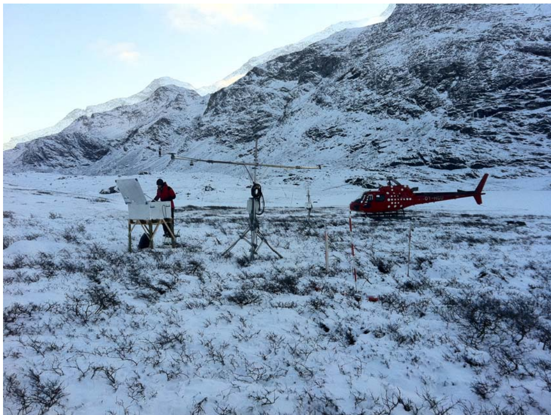
Final installation work at the Nuuk Heath site on 24 November 2011.
