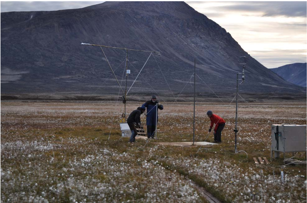
The INTERACT/ICOS construction work in the Zackenberg fen area during August 2011
